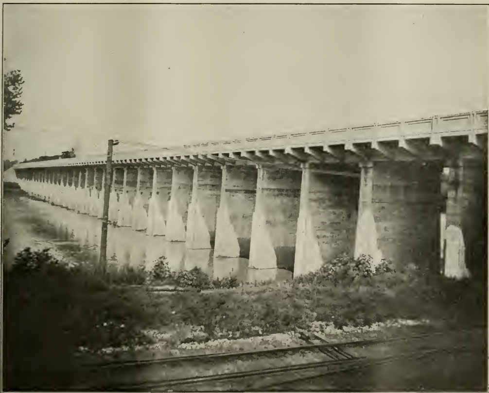
DOUBLE TRACK CONCRETE VIADUCT OVER THE DAN RIVER AT DANVILLE, VA.
